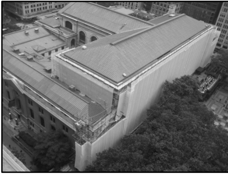
Figure 8. Scaffolds enclose west facade to avoid disruption to abutting restaurant
