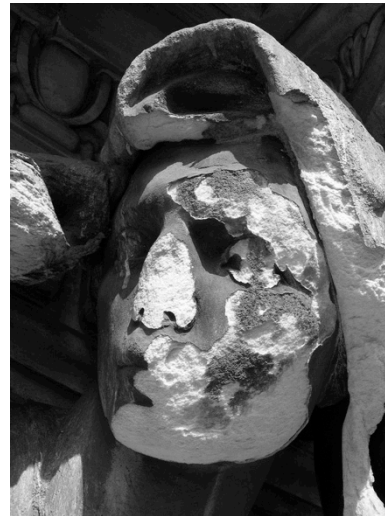
Figure 4 (above): Barnard pediment group detail showing extent of deterioration prior to treatment.
