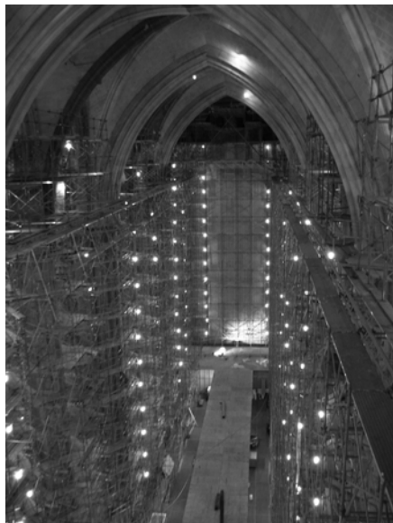
Figure 1. View of scaffolding at nave. Center aisle is open, with plywood-roofed pedestrian walkway. Plywood secured to pipe frame, visible at center rear, provides separation between nave and crossing. Photograph by the author.
