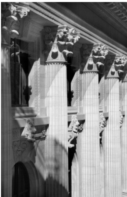
Figure 10. Detail of completed front facade
