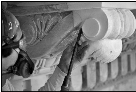
Figure 7. Marble dutchman patches were carved in place
