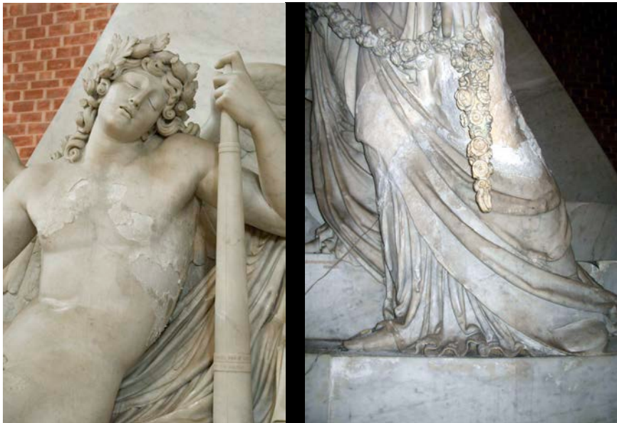
Fig. 2, 3. Details of exfoliation on the Sleeping Genius and on the womens' dresses.
