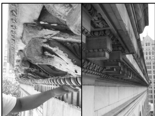
Figures 5a and 5b. Deteriorated modillions at main cornice without drip groove (left) and sound modillions at high cornice (right) with drip groove.
