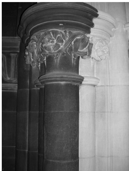
Figure 4. Detail of limestone surface cleaned by Arte Mundit adjacent to uncleaned section of stone. Photograph by Andrew Wilson.
