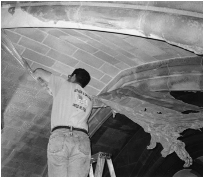
Figure 3. Removal of cured Arte Mundit in progress. Photograph by the author.
