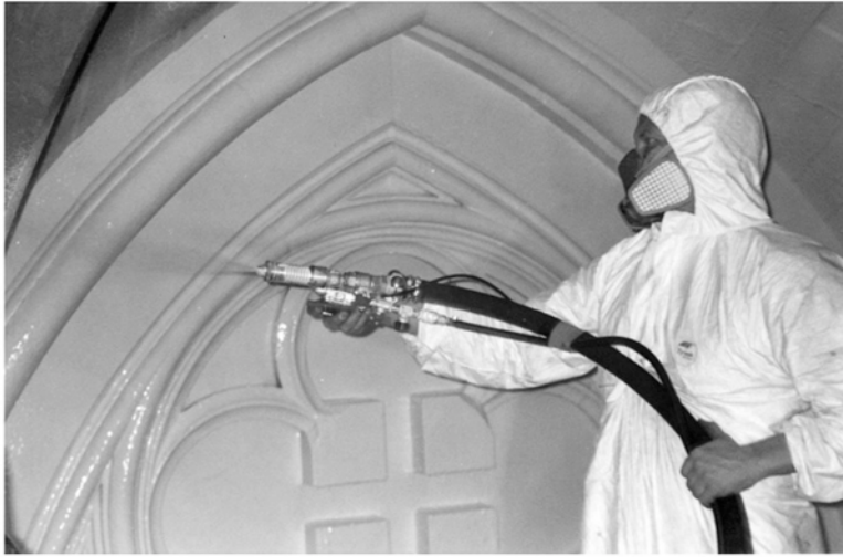
Figure 2. Spray application of Arte Mundit in progress. Photograph by the author.
