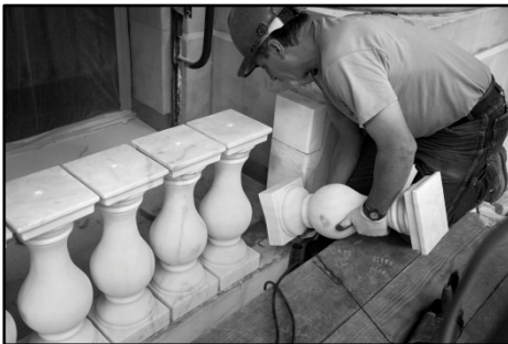
Figure 9. New turned marble balusters were installed at all balconies and parapets
