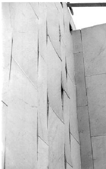
Figure 1. Bowing of marble claddings (from TEAM brochure, see also www.sp.se/Building/TEAM )
