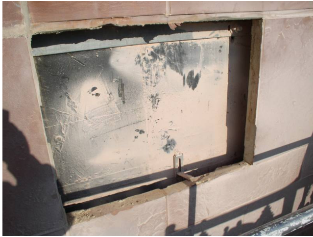
PHOTO 3 - MISSING ANCHORS
