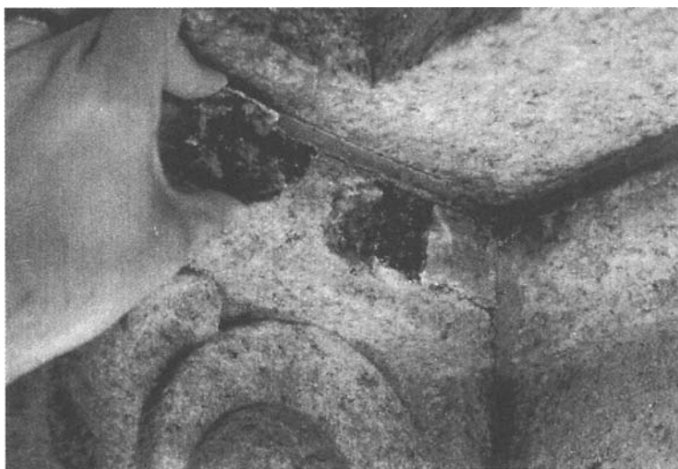
Figure 4 - Organic growth present behind incipiently exfoliated granite
