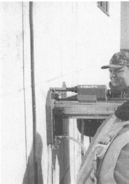
Figure 14 - Supplemental anchor mock-up, coring countersink hole for supplemental anchor head
