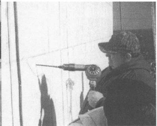
Figure 15 - Supplemental anchor mock-up, drying of anchor hole
