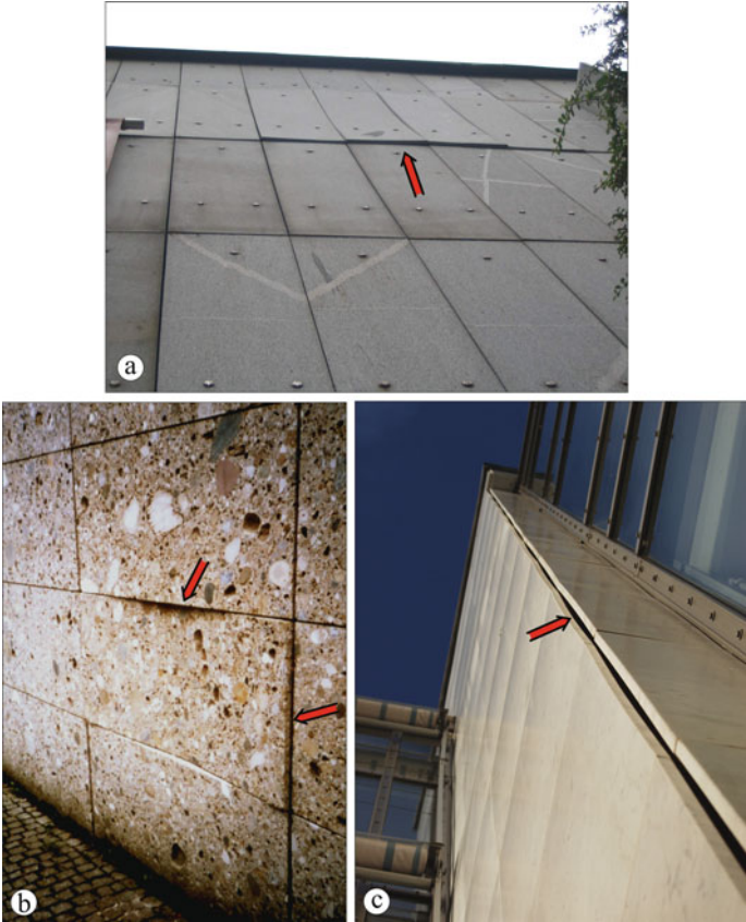
Fig. 3.78 Photos of cladding showing bowing: (a) granite (Siegesmund et al. 2008a), (b) Nagelfluh Conglomerate (after Grimm 1999), and (c) marble (Siegesmund et al. 2008b)
