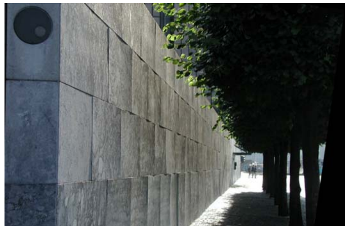
Figure 1. Bowing panels on a facade in Copenhagen.
