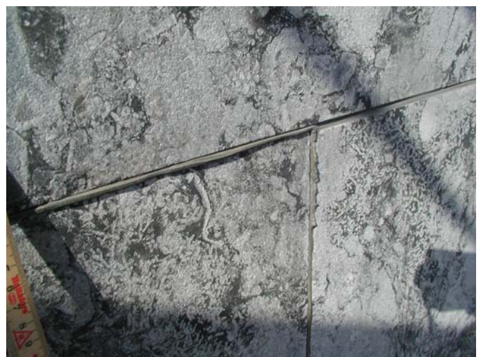
Figure 2. Expansion of panels leads to contact stresses and compaction of joint material, which can be squeezed out.
